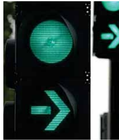
Traffic signalling upgrades
